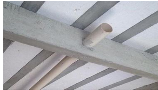
Figure 1 Concrete beams with openings
