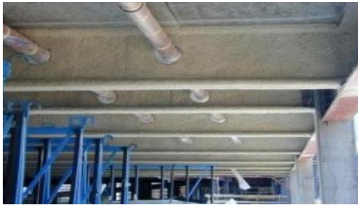
Figure 1 Concrete beams with openings
